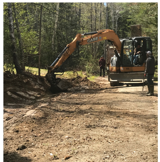
Ditch work on South Shore Colony Road
