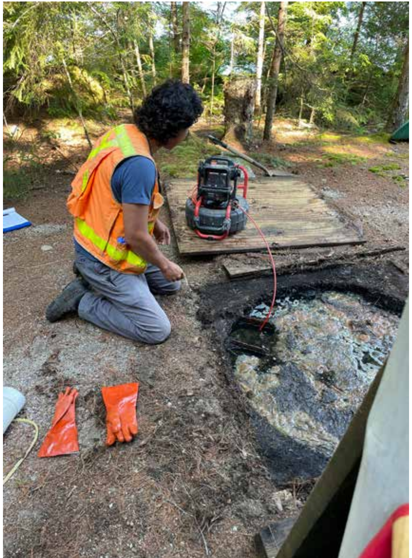
Figure 11. Septic system inspection.
