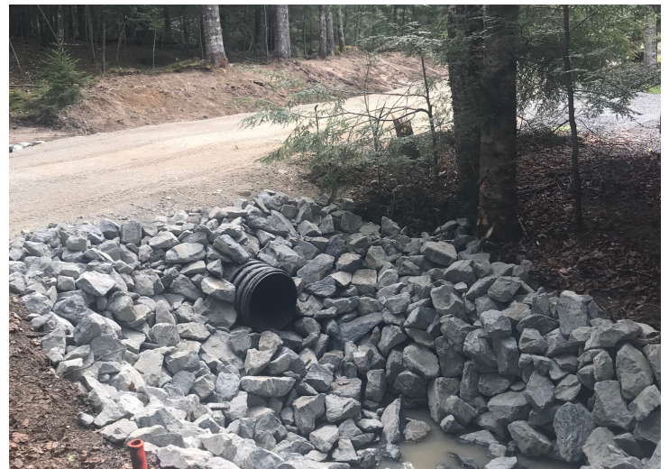
New culvert and plunge pool on South Shore Colony Road.
