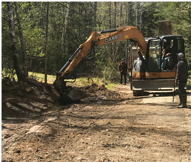
Improving the drainage ditch on South Shore Colony Road
